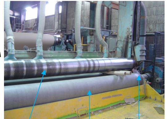
Rider Roll. Winder Drum. Cardboard Cores. (cores indicate position of employee legs at time of incident)
